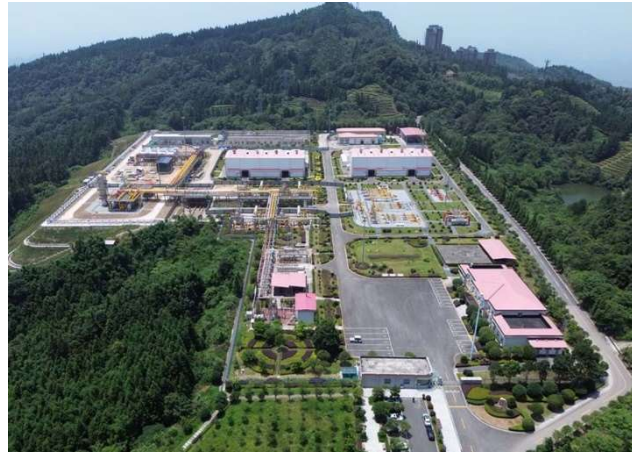
Fig. 1 Aerial view of Xiangguosi gas storage injection and production station
