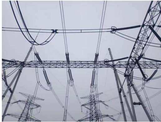
Figure 3. Hoisting site environment
