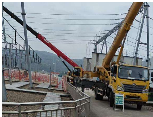
Figure 4. The crane is in place
