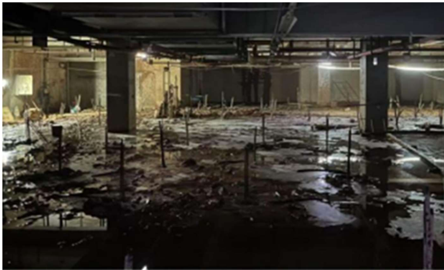
Fig.1 Reinforcement Construction Photograph
