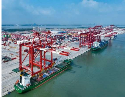
Fig. 4 River and sea vessels berthing on the same side at Nansha Phase IV Fully Automated Terminal, with transshipment via the front yard
