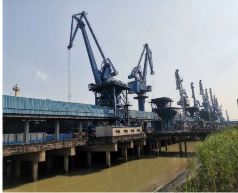
Fig. 2 Non-adjacent arrangement of river and sea vessel berths, with loading and unloading connected via belt conveyors
