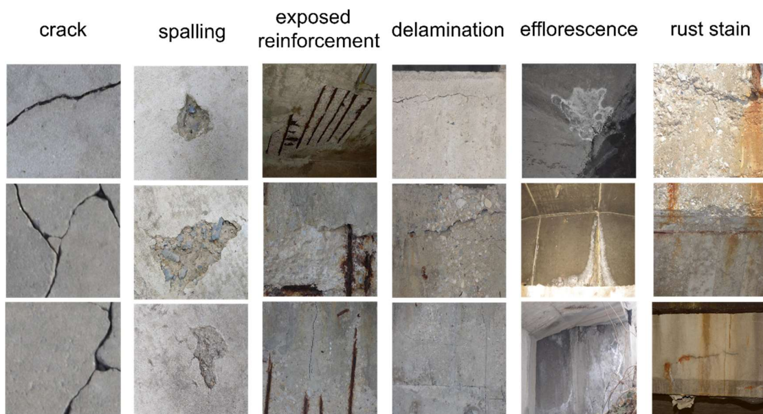
Figure 4. Types of Building Surface Defects
