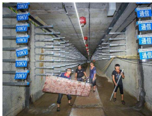
Fig. 1 Power utility tunnel construction
