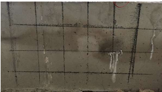
Figure 1. Temperature cracks
