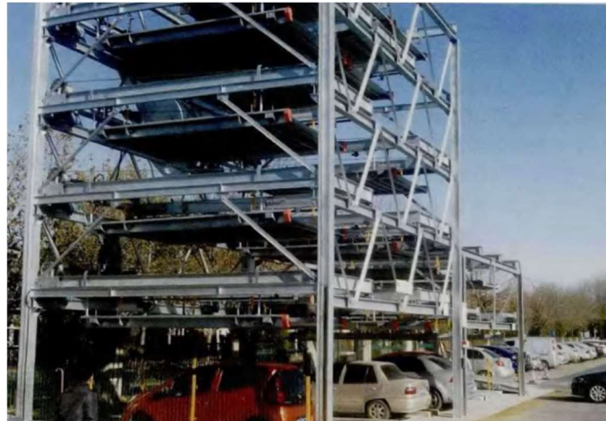
Figure 2. Traditional Steel Frame Parking Structure
