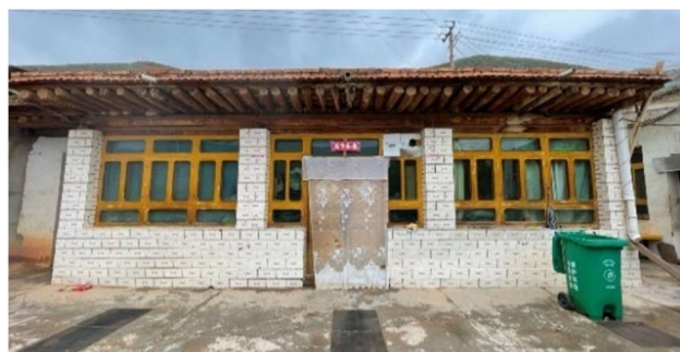
Fig. 2 Main elevation view of the house
