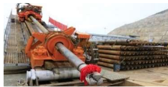
Fig. 2 Horizontal Directional Drilling
