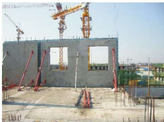
Fig. 2 Support frames underneath assembled engineered laminated panels [15]
