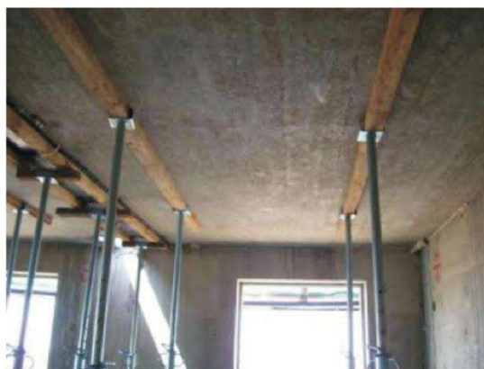
Fig. 1 Support frames underneath assembled engineered laminated panels [15]
