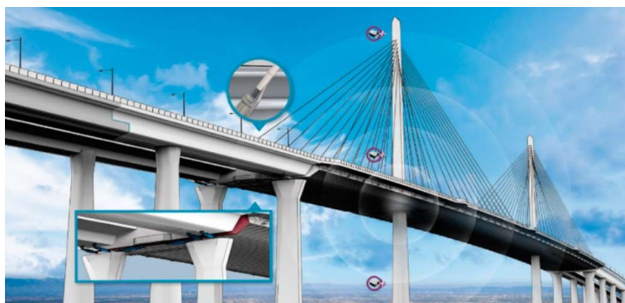
Fig. 2 Sensors mounted on the outside and middle of the main beam
